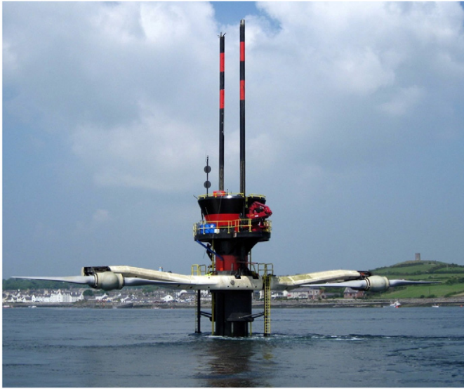
Fig. 1. Twin-turbine system with horizontal turbines (courtesy of Peter Frankel).
